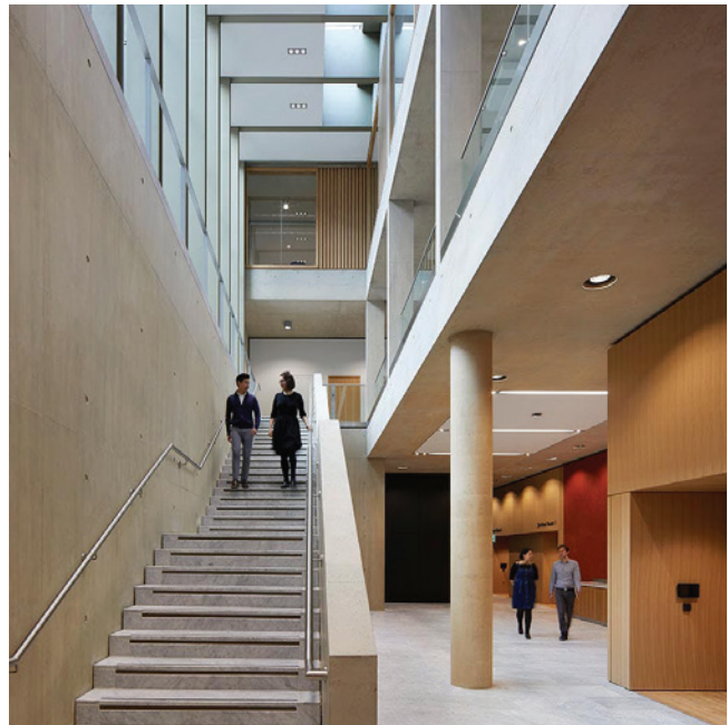
The Simon Sainsbury Centre at Judge Business School, Cambridge uses an innovative natural ventilation system, in combination with the thermal mass, to minimise energy consumption. Architect: Stanton Williams; Structural Engineer: AKT II. Image © Hufton and Crow.
